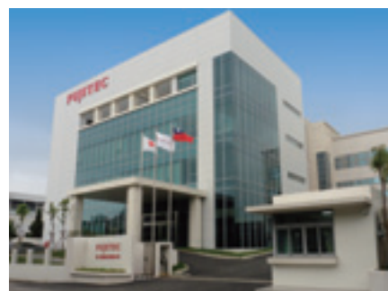
Renovation of the Hsinchu Plant completed at Fujitec Taiwan Co., Ltd. (March 2016)
